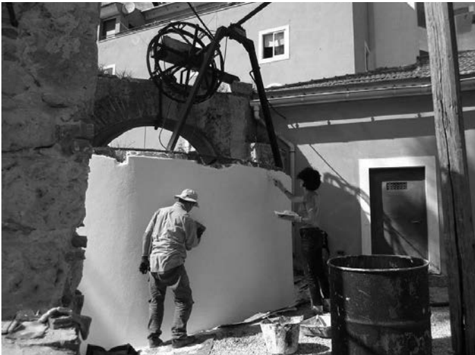
Fig. 4: Learning how to restore a noria with traditional whitewash techniques. Photo: Author, 2015.
