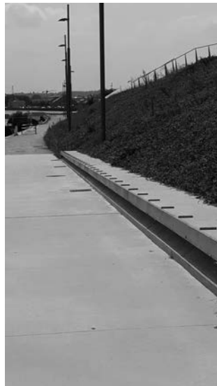
Fig. 4: Pig's ears deter unwanted skateboarding on concrete blocks in the Jardin du Musée des Confluences, Lyon (France). Photo: Smaniotto, 2018.
