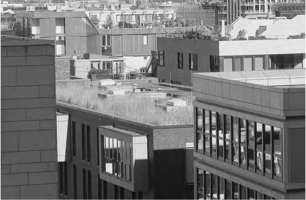
Fig. 4: Roofscape in Hamburg, Hafencity. Green roofs offer sites for vegetation without requiring additional space. Extreme conditions regarding climate, soil and water-supply pose challenges, to them vegetation technology has to find solutions. Photo: Westerholt, 2017
